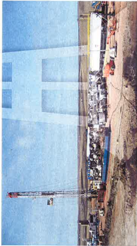
Fracture stimulation operations at the Gene #1-22H well
